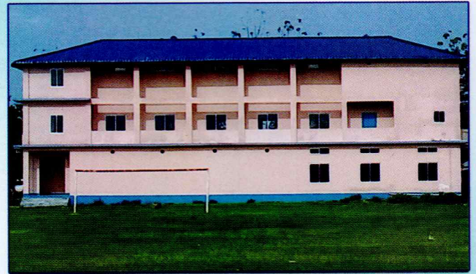
Multi-purpose Community Hall of the College.
